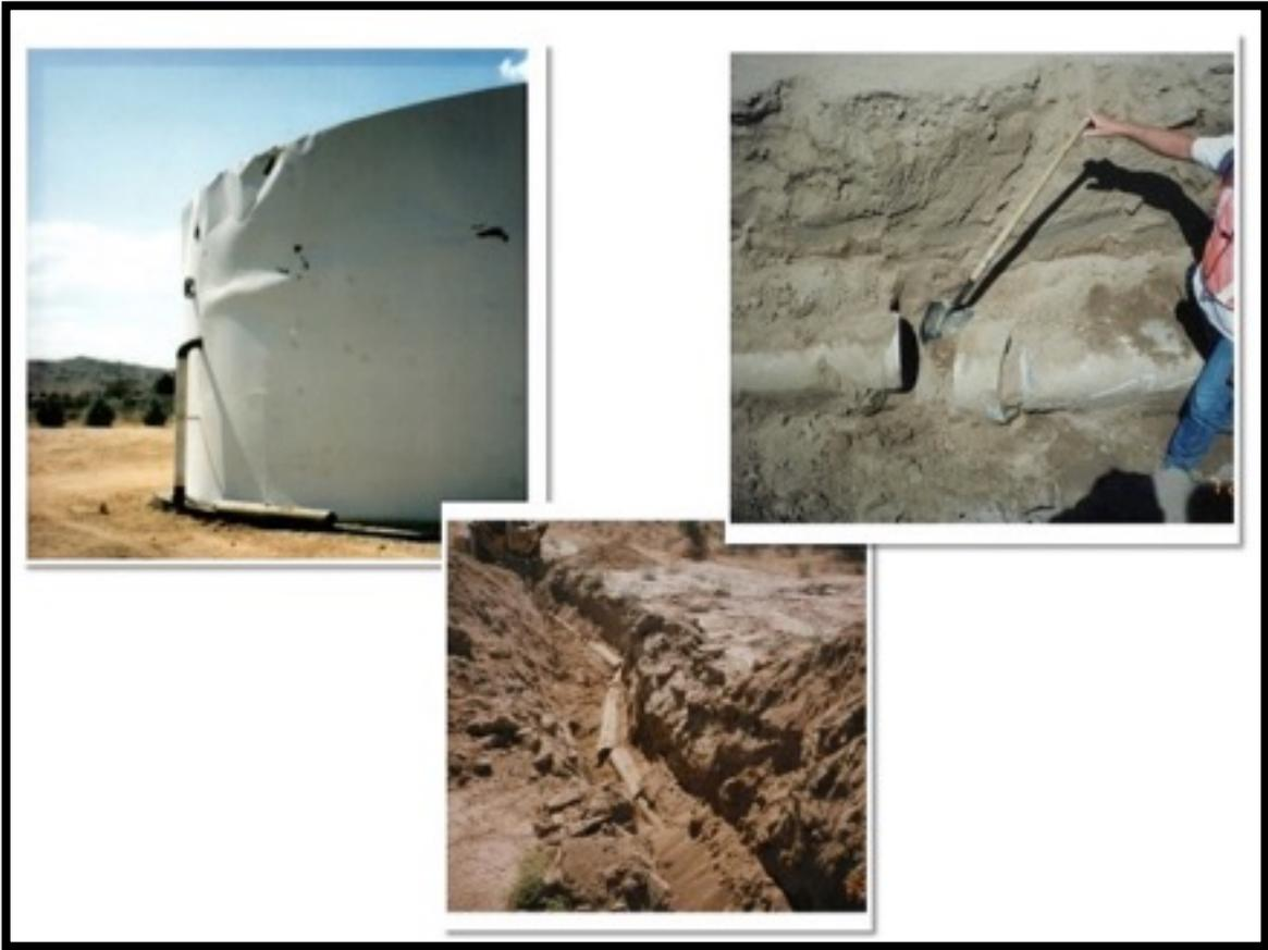
**Figure 2 Examples of Earthquake Damage to Water Utility Facilities**
