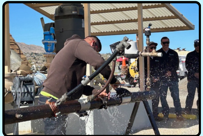
Leak repair demonstration-- stand back!
