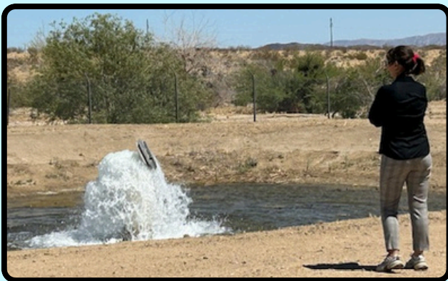
Observing Well 14's periodic flushing
